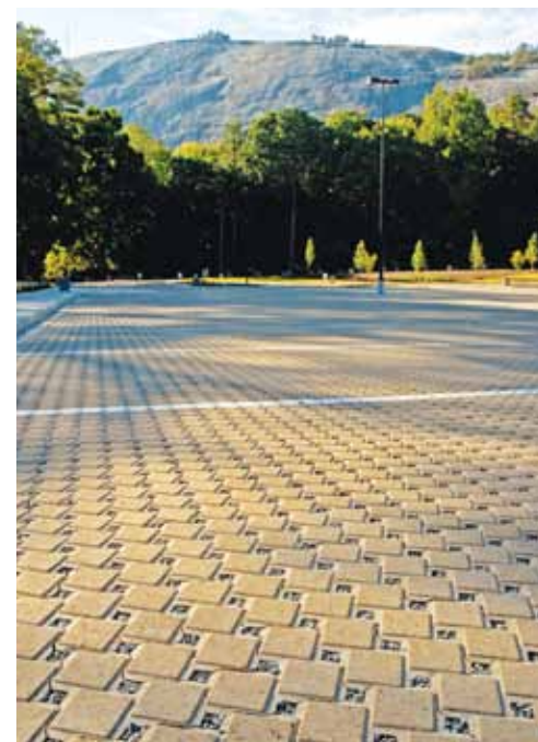
The parking lot at Stone Mountain Park is a highly successful example of pervious paving.
