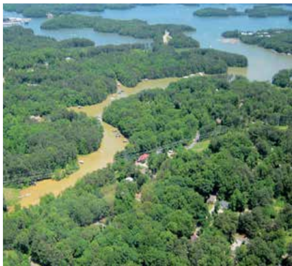
A breach at the Lake Alice dam dumped tons of sediment into Lake Lanier.
