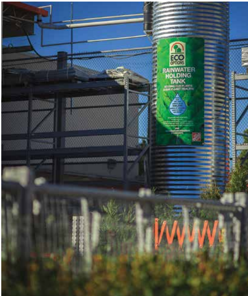
Each rainwater tank helps The Home Depot save 500,000 gallons per year.
