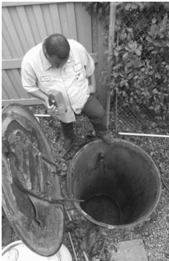
Photo by John Covington/Savannah Morning News A wastewater vacuum truck operator inspects a trap which has collected grease from Savannah's sewer system.
