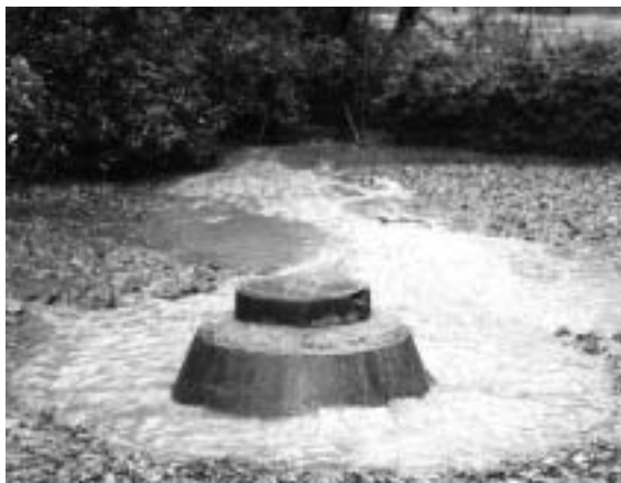
Raw sewage spilling out of a manhole into the River is a good reason to get involved with Riverkeeper's HOTLINE!
