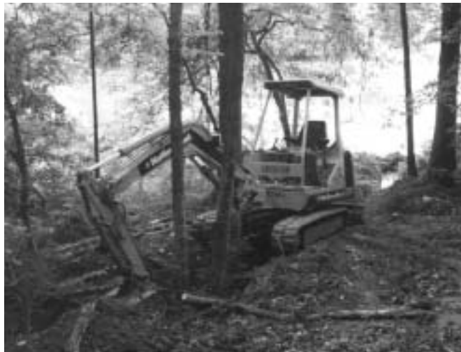
Bulldozer digs ditch for Eagle Golf Course water withdrawal.
